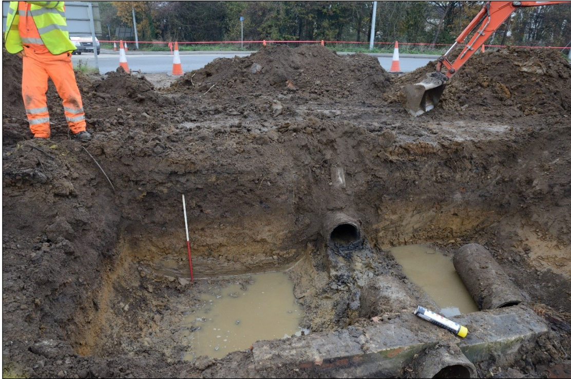
Plate 3: Area C, Section 1, looking northwest; 1m scale
