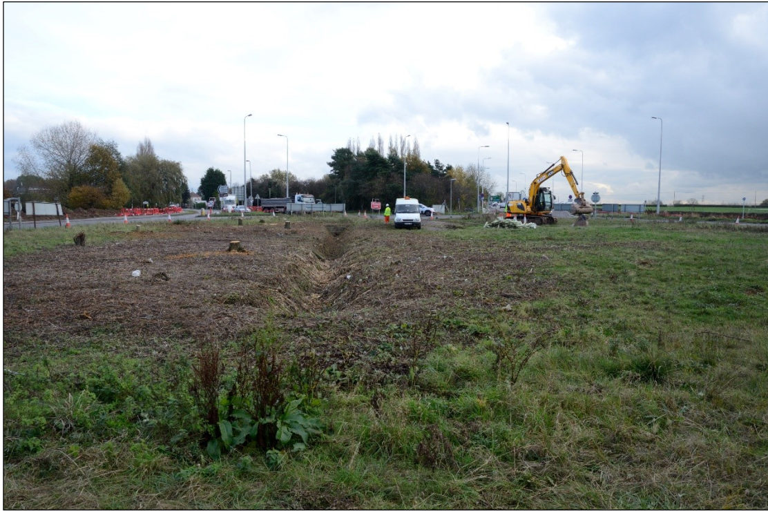
Plate 1: Initial ground clearance on the island at Dodwells Roundabout, looking east
