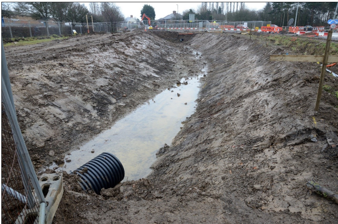
Plate 8: New drain northeast of the roundabout (Area D), looking southeast
