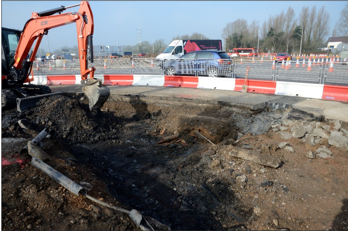
Plate 13: Work in progress, east side of the roundabout, looking c. west
