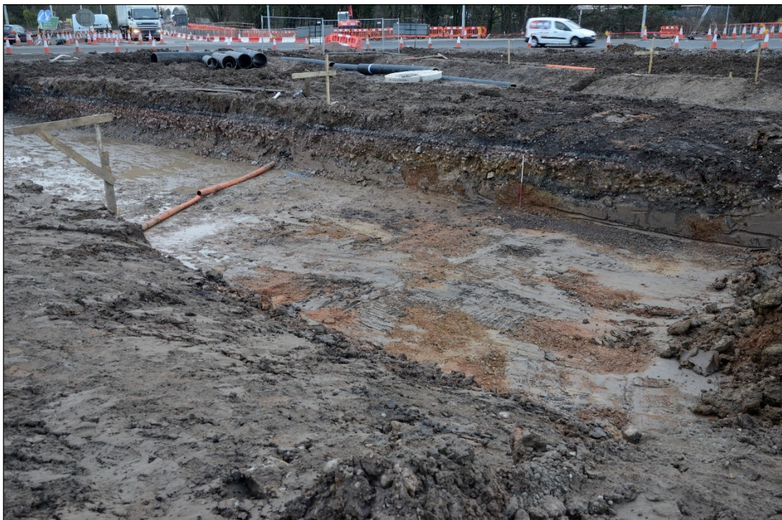
Plate 6: Excavation for water storage feature (Area A), looking northwest; 1m scale
