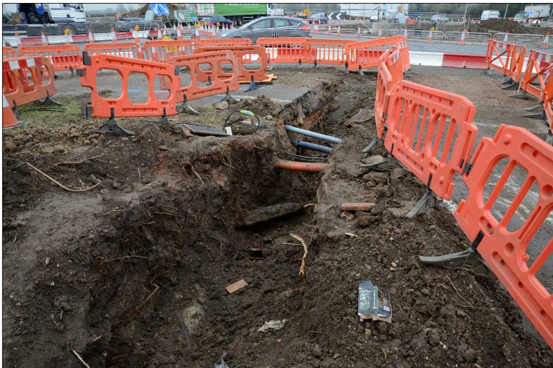
Plate 12: Work in progress, east of the roundabout, looking c. west
