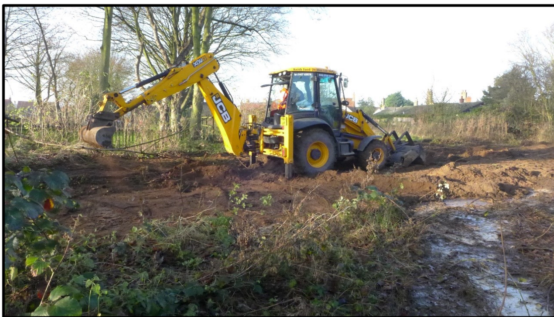
Plate 2: Machine excavation of Trench 3 in progress, looking northwest
