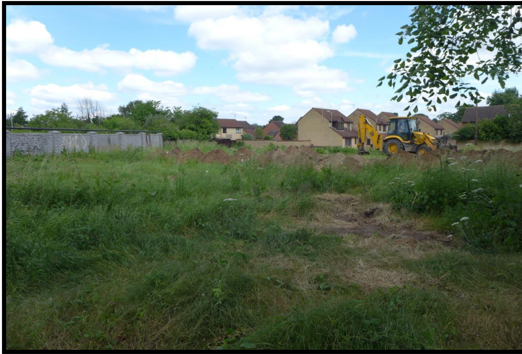
Plate 3: General view to the development area looking north
