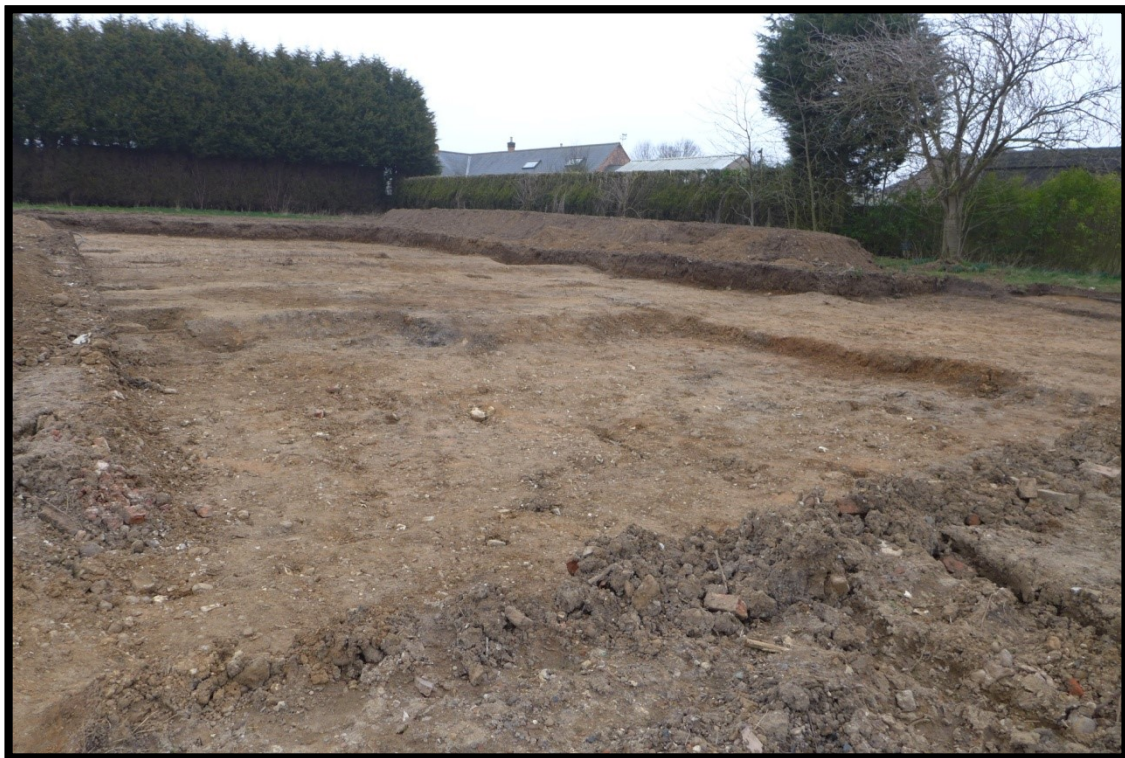
Plate 2: View of Area A under excavation facing east.
