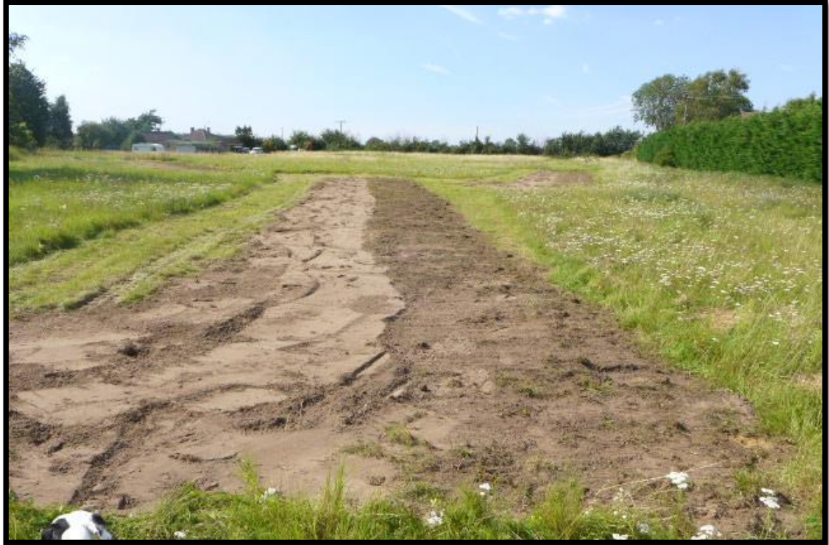
Plate 5: General view of the development area looking southwest, showing backfilled Trench 6
