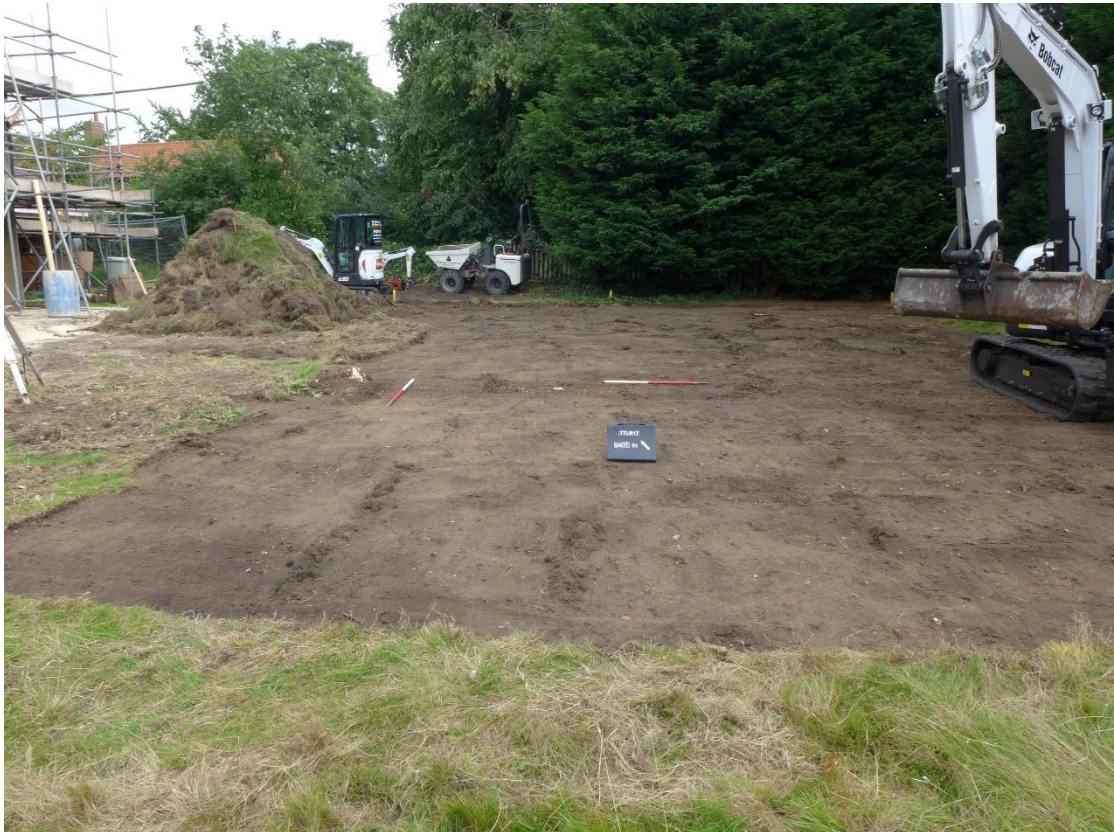
Plate 2: Car park area after turf stripping, looking northeast, Scale 1m
