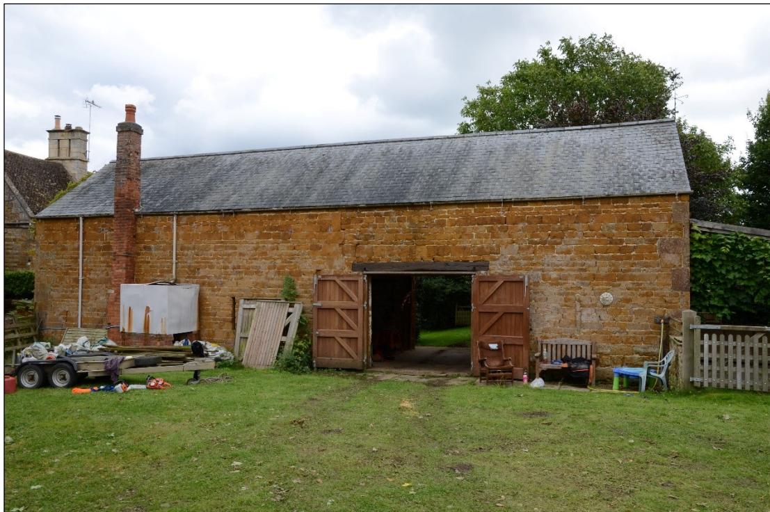
Plate 10: Northwest facing elevation, looking c. southeast
