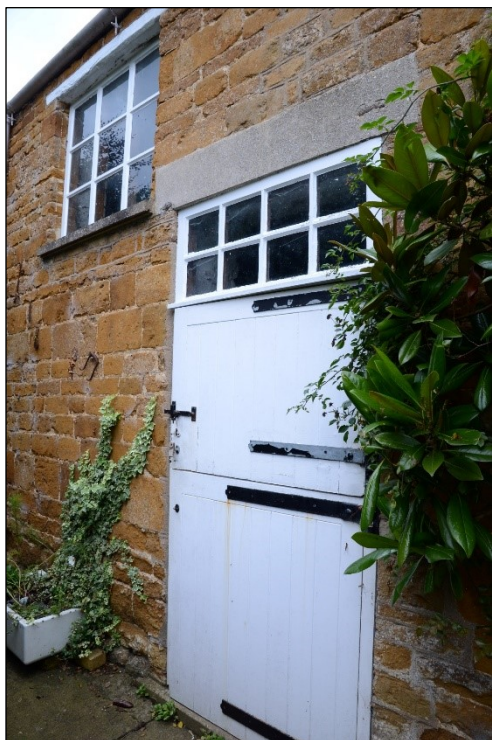
Plate 7: Door and former pitching door (top left) in the southeast facing elevation, looking west
