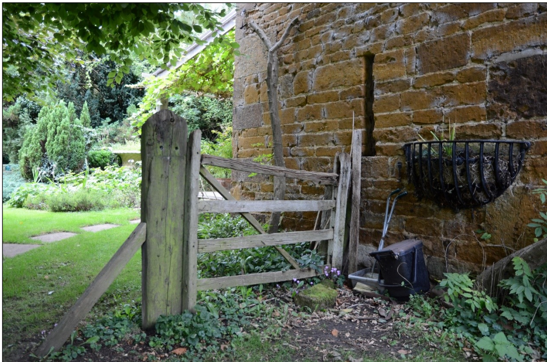
Plate 6: Southwestern end of the southeast facing elevation, looking west
