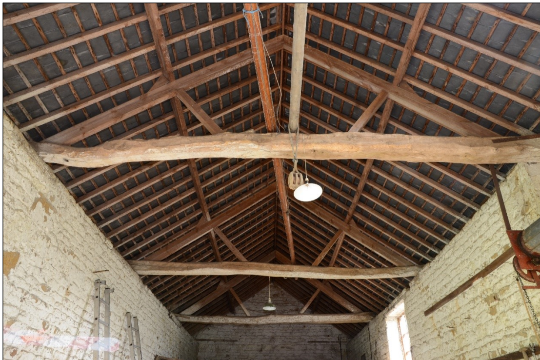
Plate 17: Roof of the barn, looking northeast from between the doors
