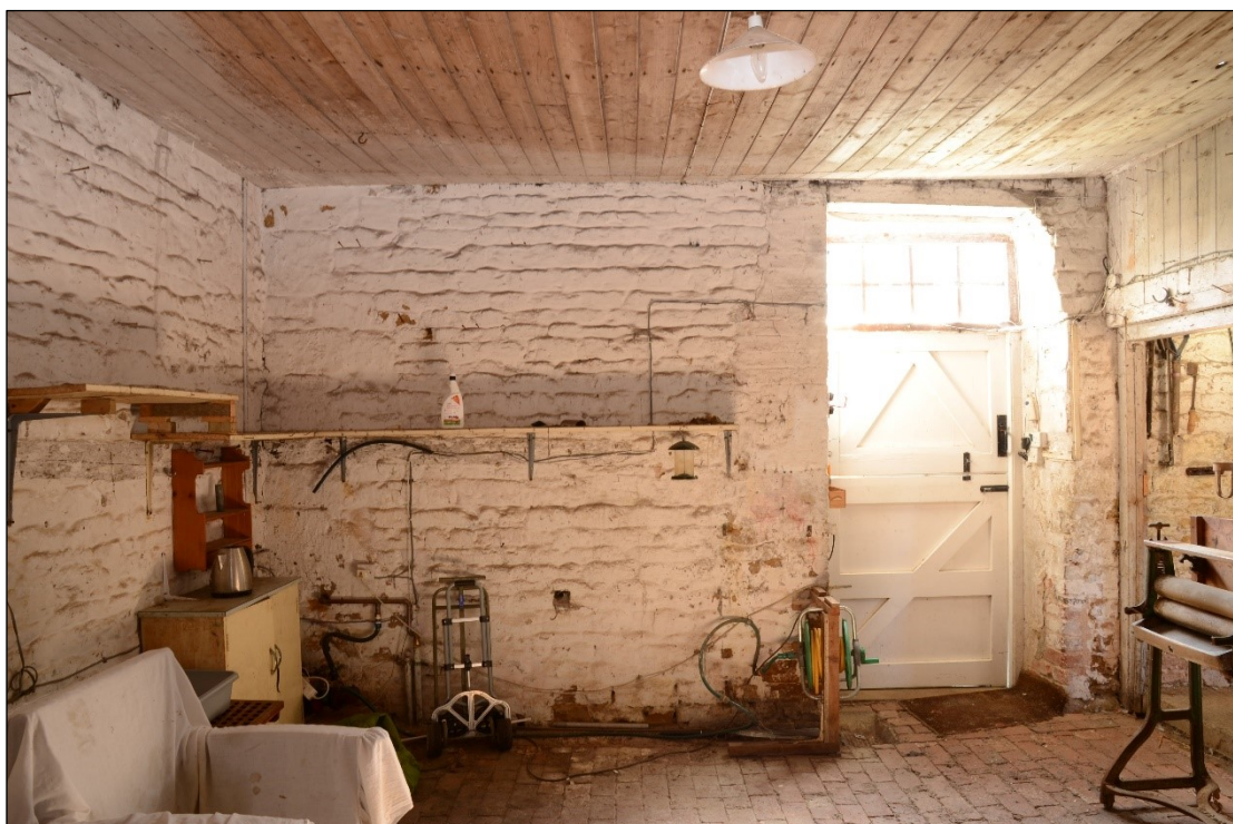
Plate 26: Southeastern side of the washroom, looking southeast
