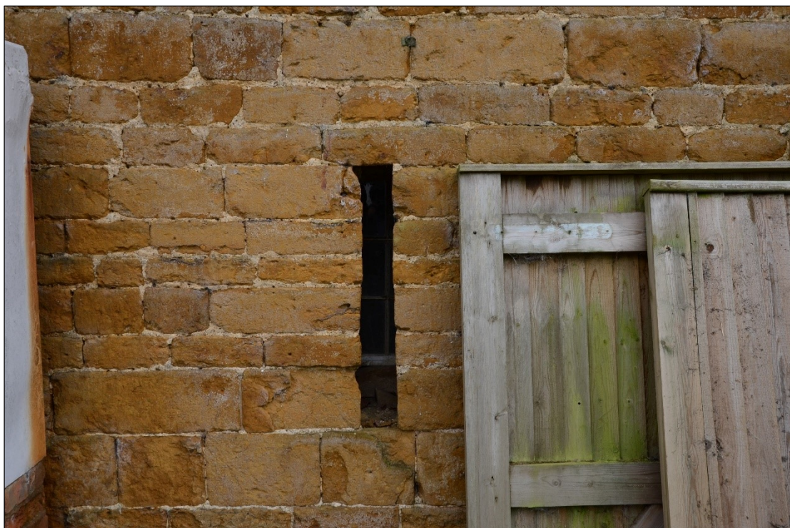
Plate 13: Vent in the northwest wall, northeast of the door, looking southeast
