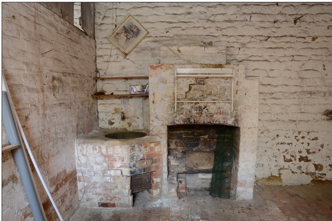
Plate 25: Detail of brick copper and fireplace in the washroom, looking northwest
