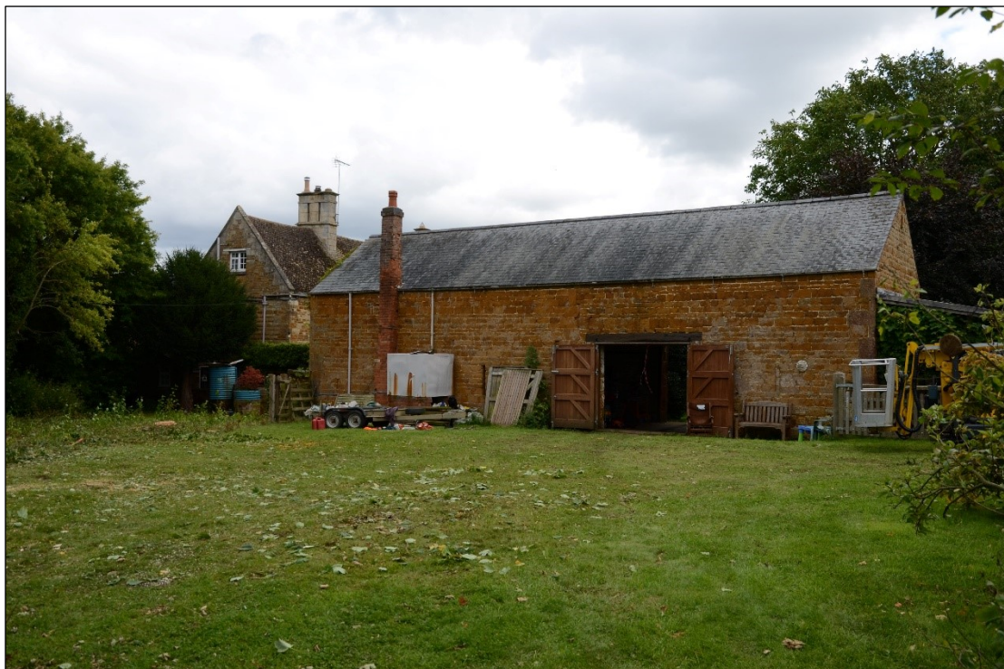
Plate 3: General view from the north-northwest
