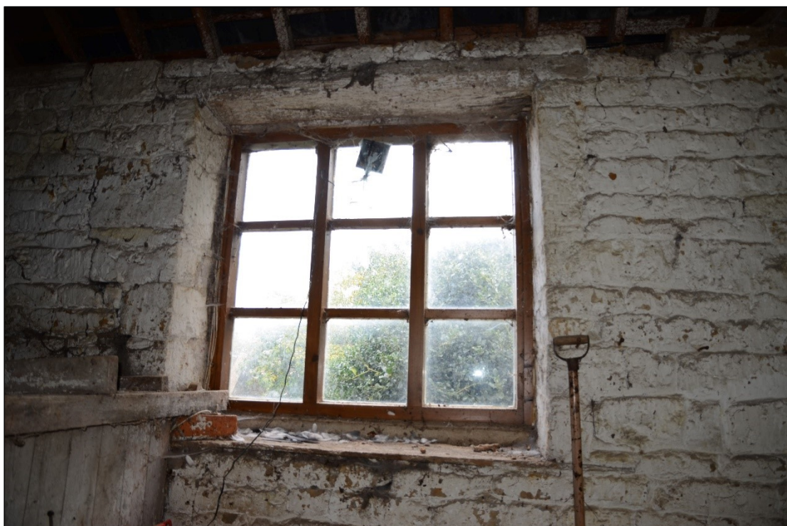
Plate 18: Former pitching door in the southeast wall, looking c. southeast
