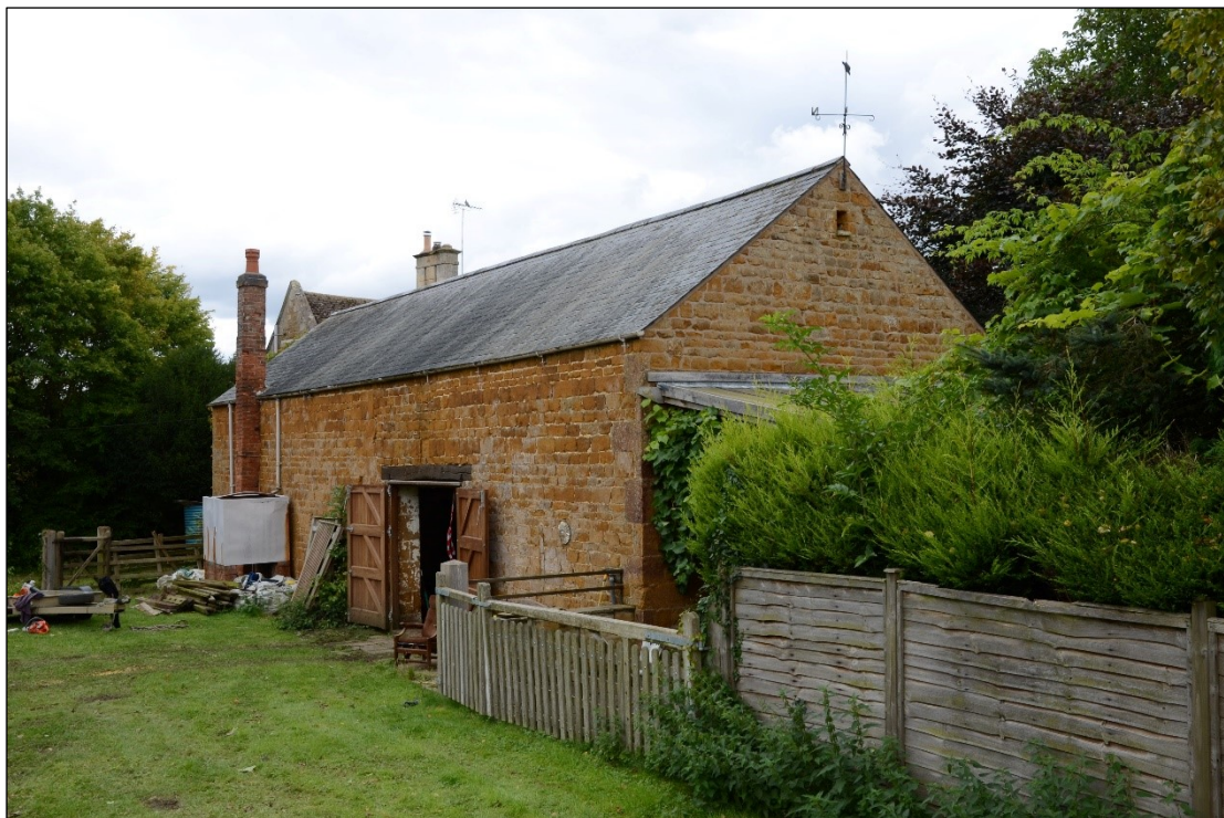
Plate 9: Northwest and southwest facing elevations, looking c. east-northeast
