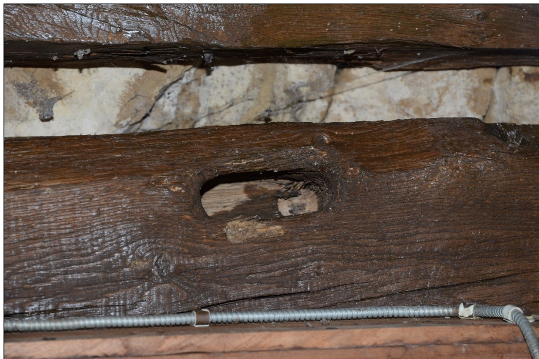
Plate 23: Recess midway along lintel over the northwest door, from directly below (northwest at bottom)
