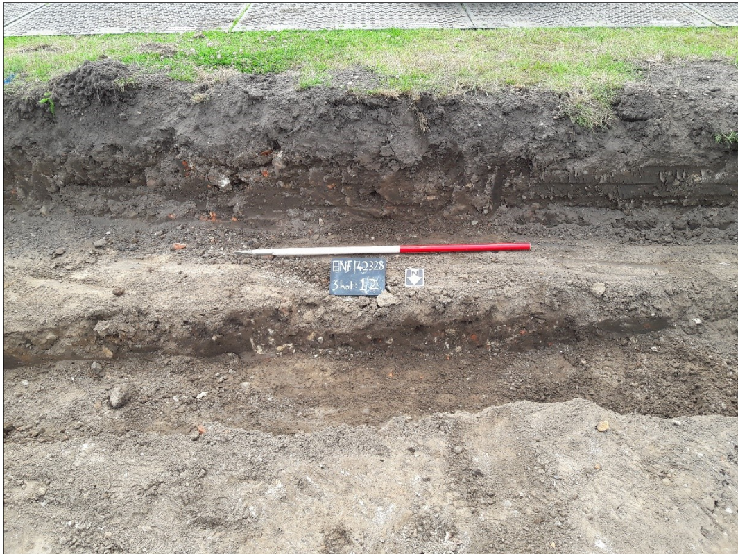
Plate 6: Section 4 at the southern edge of the stripped area, showing wall foundation or robber trench [010] (up and left of 1m scale), looking south
