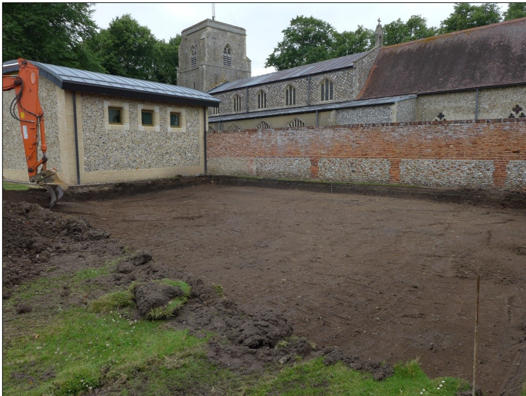
Plate 2: Stripped area in the northeastern part of the site, looking northwest
