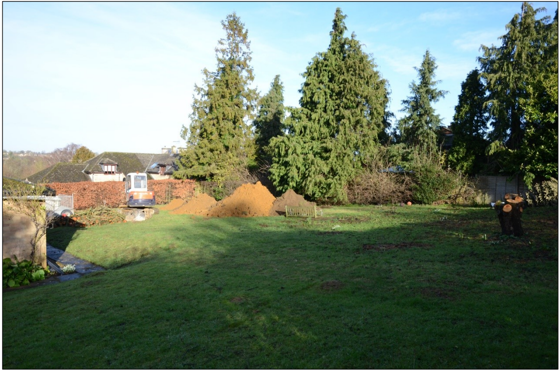
Plate 1: General view of trial trenching, looking north
