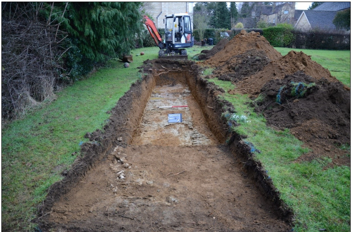
Plate 2: General view of trench, looking southeast; 1m scale
