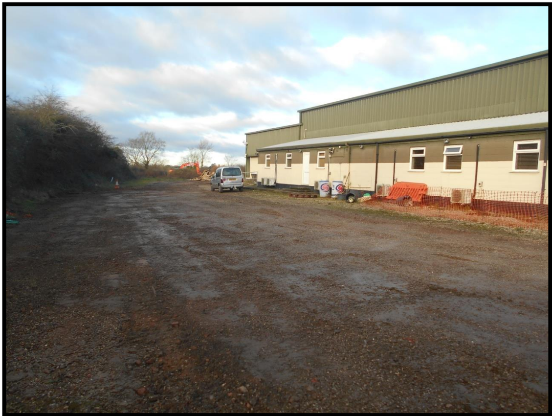
Plate 6: View of the southeast side of Area C facing west
