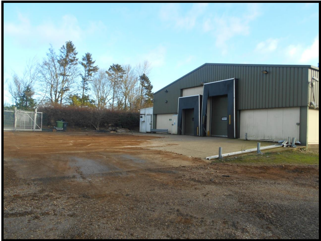
Plate 7: View of concrete pad on west side of building in Area C
