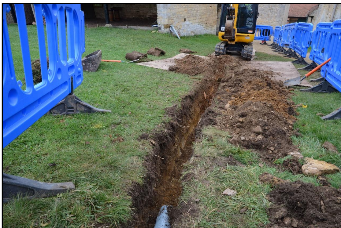
Plate 6: General view of trench excavation approaching farmyard, looking southeast
