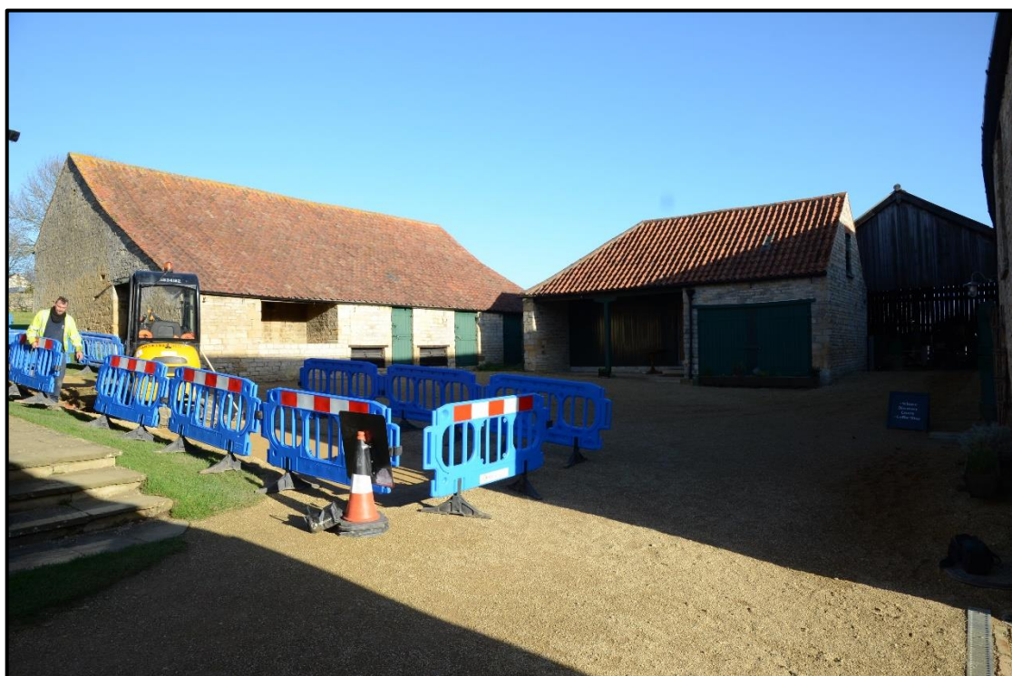
Plate 8: General view showing south of trench in farmyard, looking northeast
