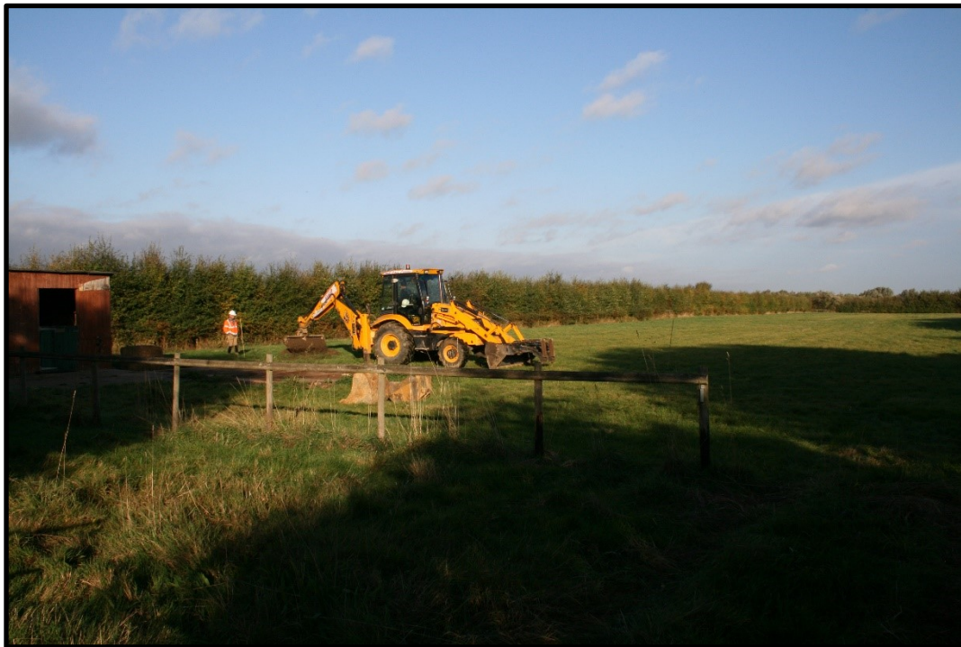
Plate 1: General view of the site, looking north-west
