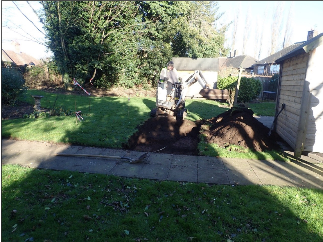
Plate 1: Excavation of Trench 1 in progress, looking north.
