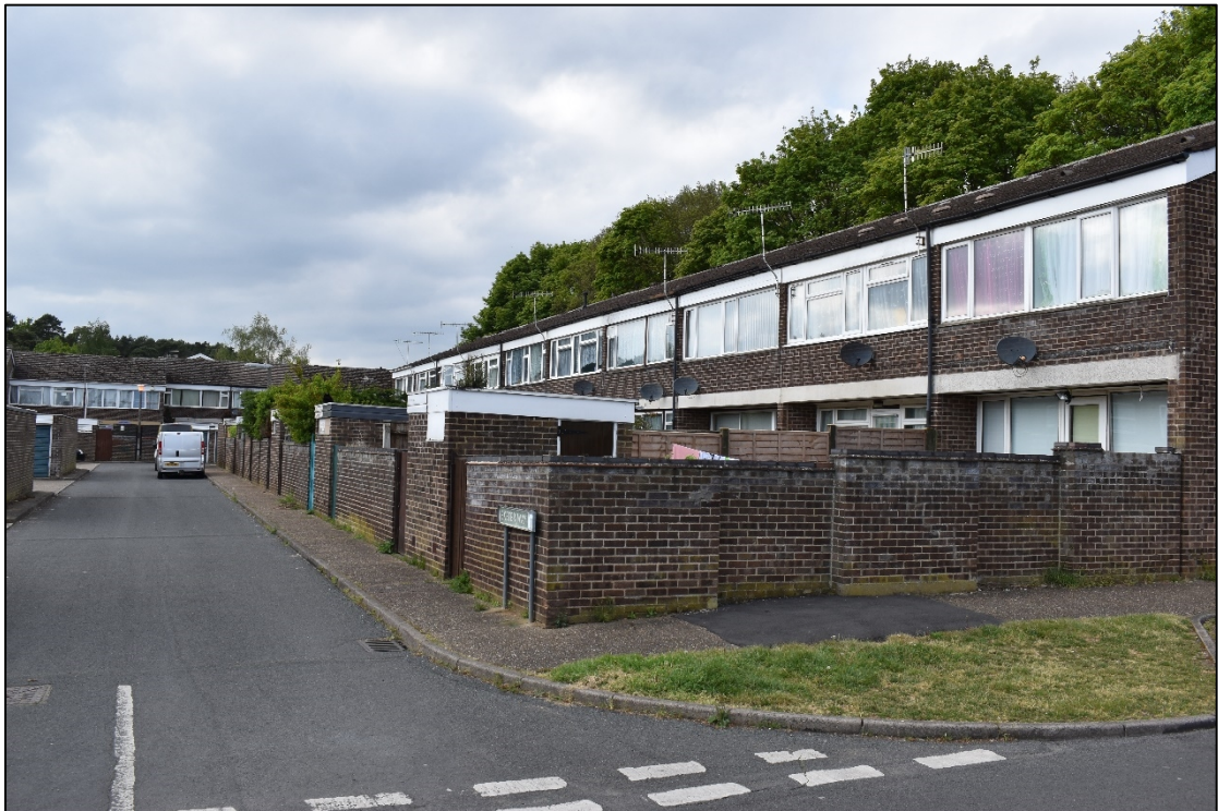
Plate 3: Two storey housing on Exeter Road
