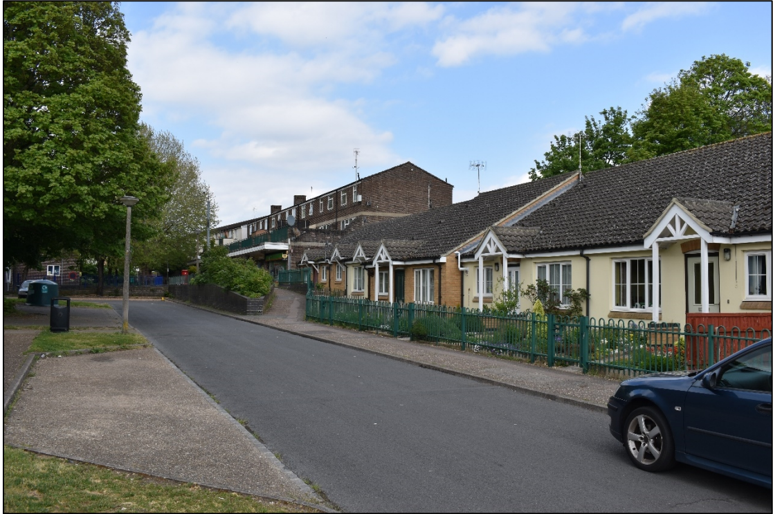
Plate 6: Bungalows on Exeter Road
