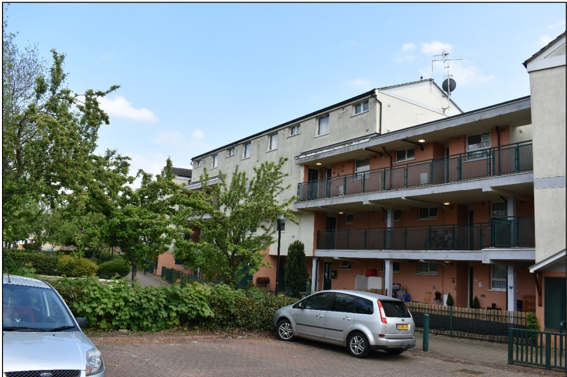
Plate 7: Flats on Salisbury Way
