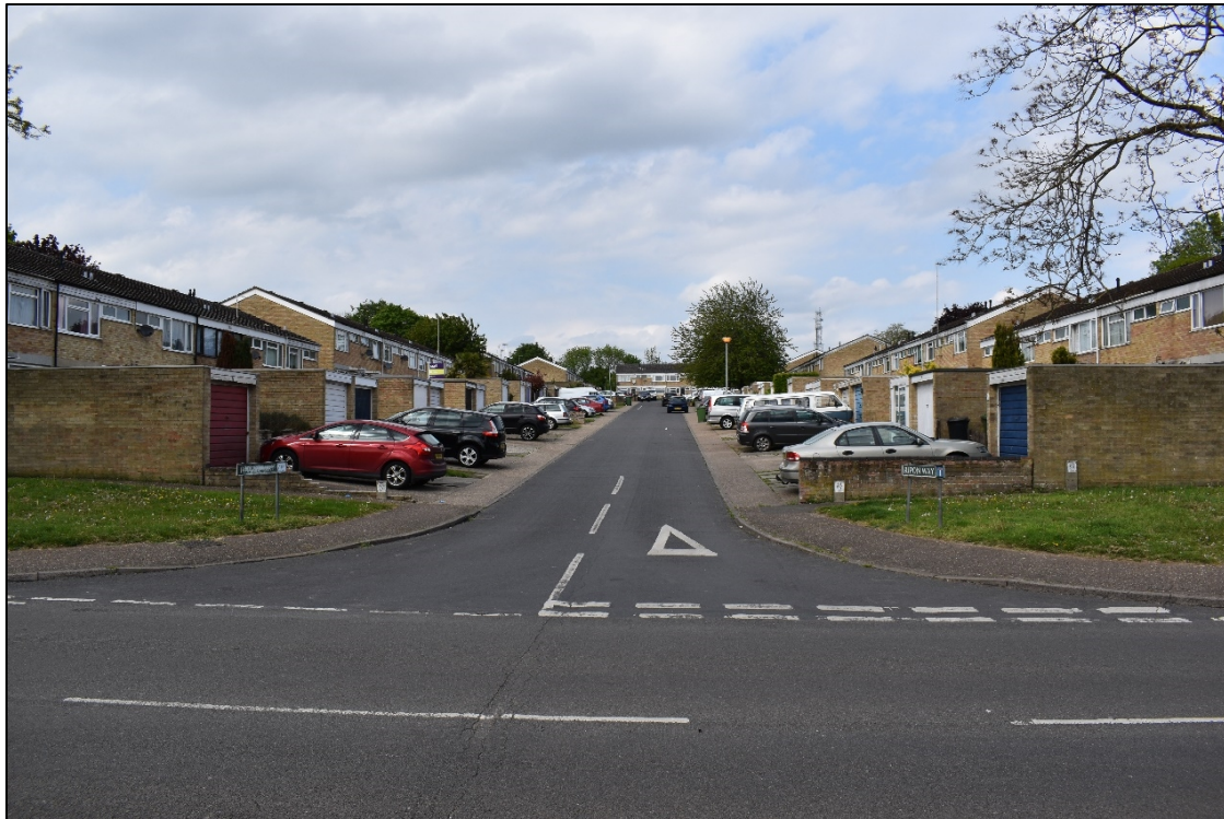
Plate 1: Two Storey housing on Ripon Road
