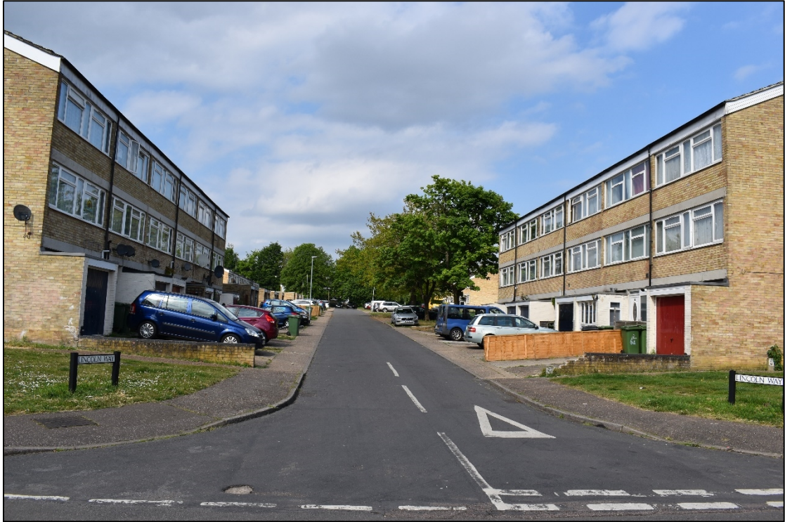
Plate 2: Three storey housing on Lincoln Way
