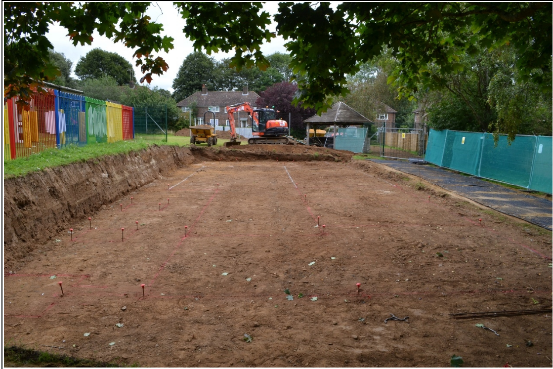
Plate 1: Area A, looking east north-east
