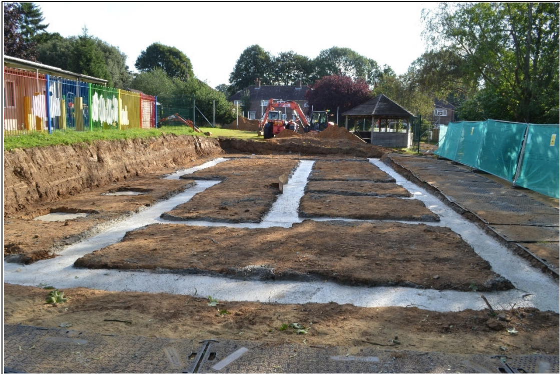
Plate 5: Area A. Completed excavations, looking west south-west
