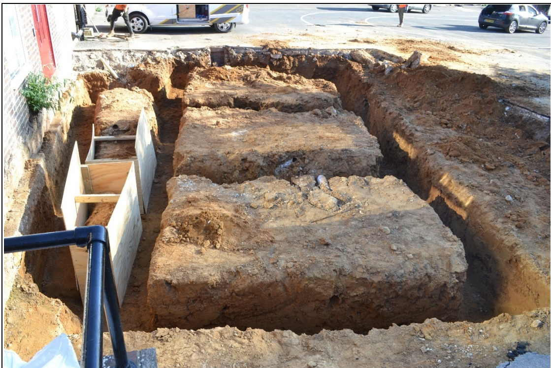
Plate 8: Area B. Completed excavations, looking south
