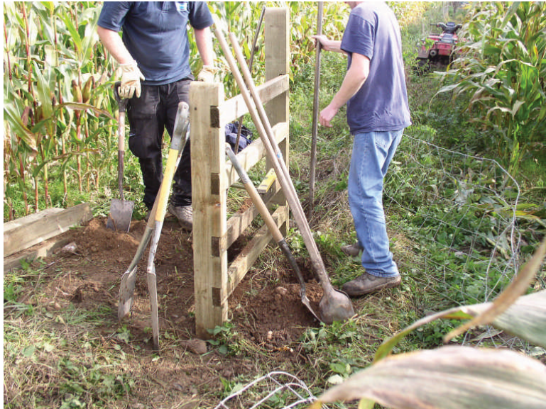
Photo 2: Stile B – new stile frame in place
