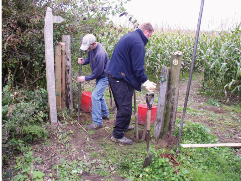
Photo 1: Stile A – post holes under excavation
