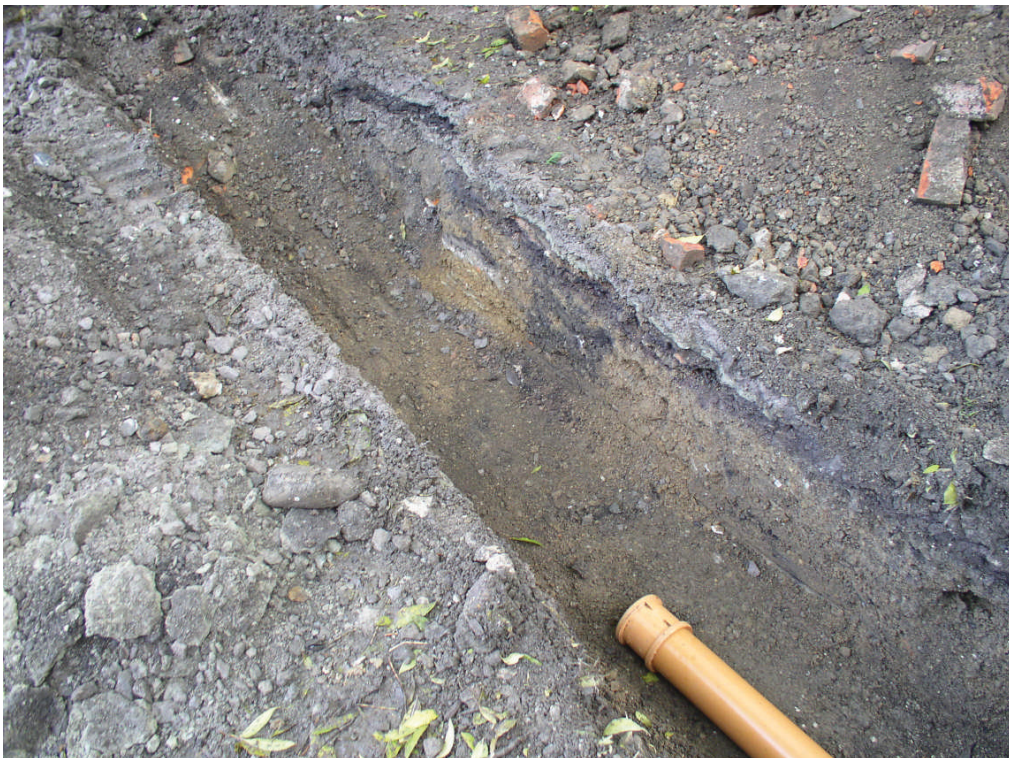
Photo 2: The new drain trench north from the Miners' Dry, looking northeast
