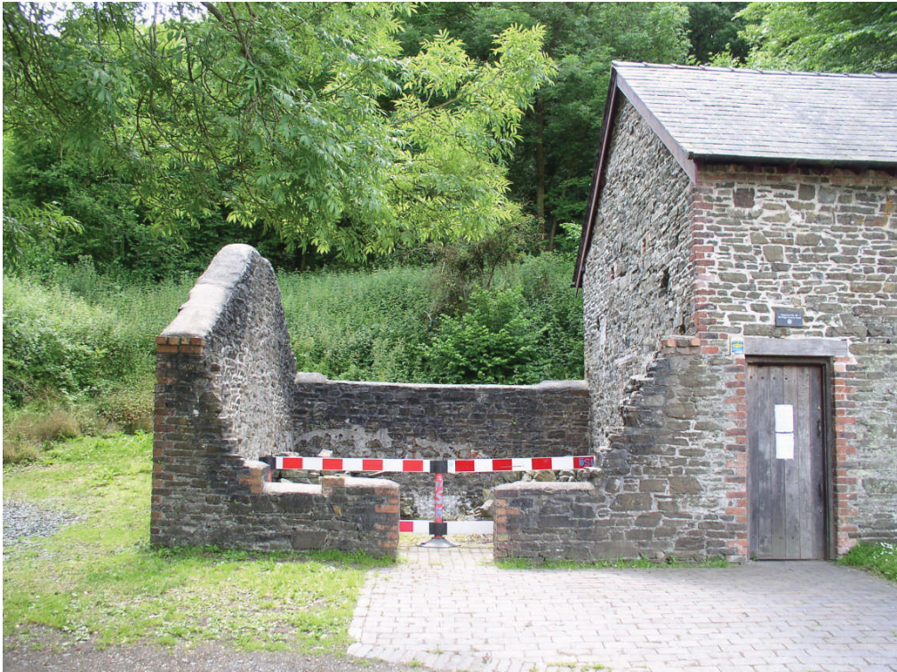
Photo 1: The Miners' Dry annexe, before conversion, looking south
