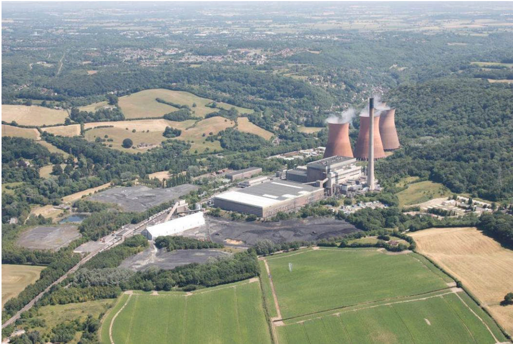
Photo 16: Buildwas power station; the site of the former power station (HER 06710) is at bottom left
