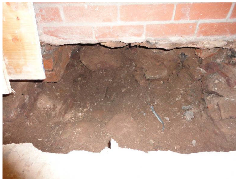
Photo 2: Test pit B, looking north
