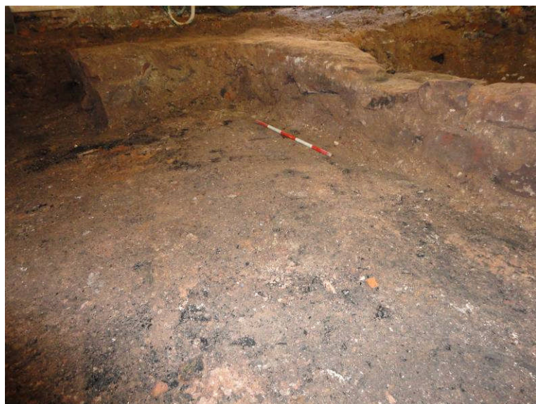
Photo 3: Wall 25 in area M, looking northwest; scale 0.5m
