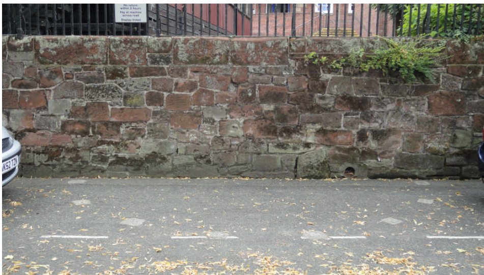
Photo 3: The site of the New Work tower (HER 01096), looking south
