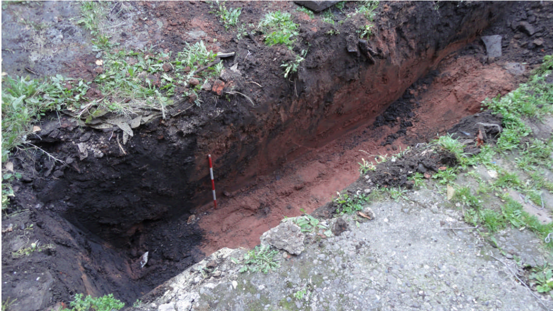
Photo 1: The foundation trench, showing pit 4, looking south
