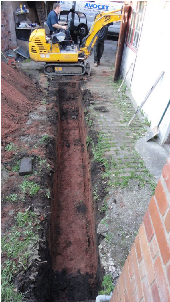
Photo 2: The foundation trench, looking southwest
