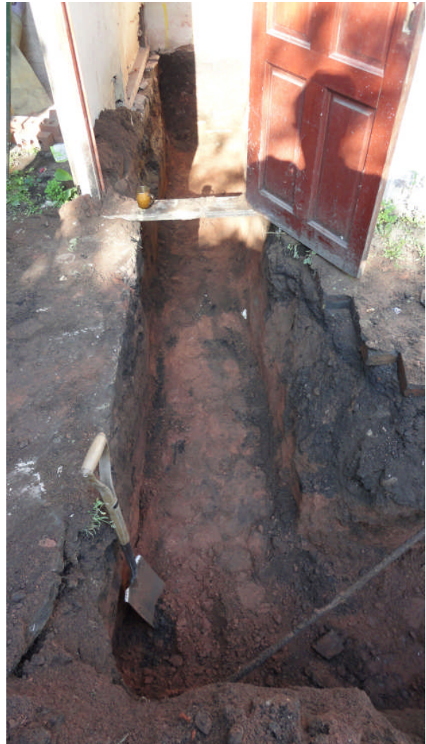
Photo 3: The foundation trench looking northwest
