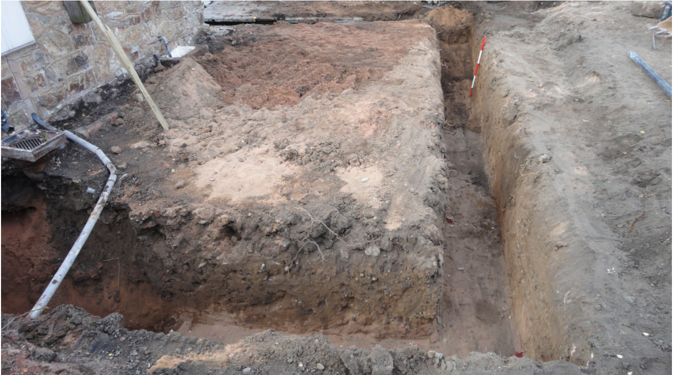
Photo 2: The deposits in the foundation trenches, looking north
