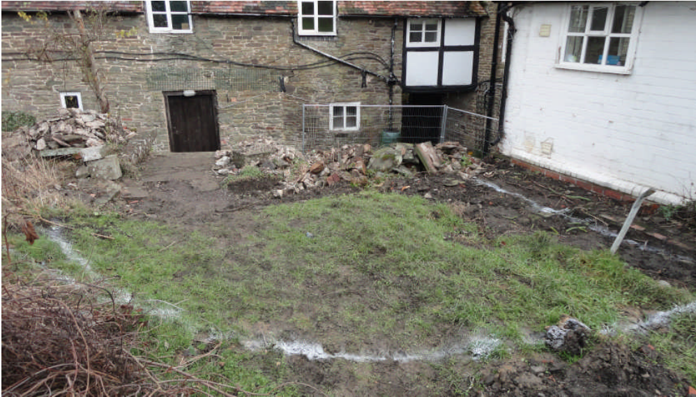
Photo 1: The study area looking northeast, before excavation
