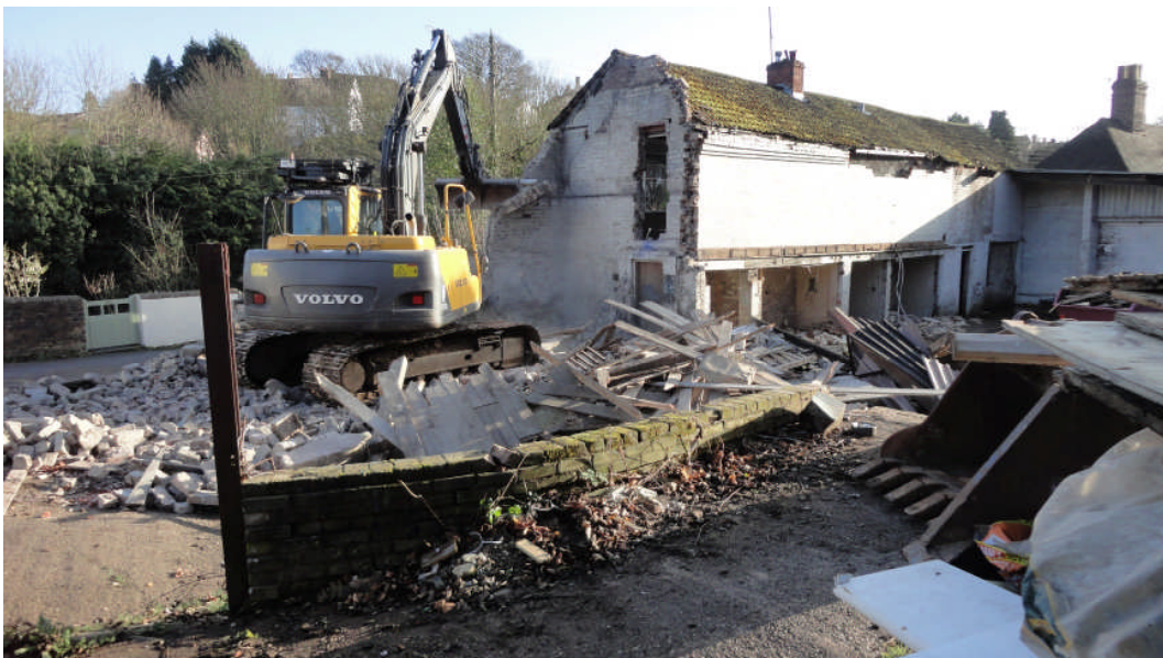
Photo 6: Demolition work in progress, looking southeast
