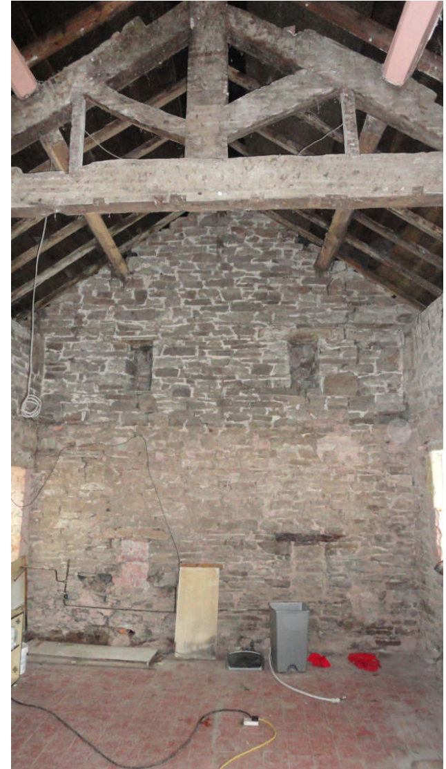
Photo 6: The E wall, interior elevation looking W
