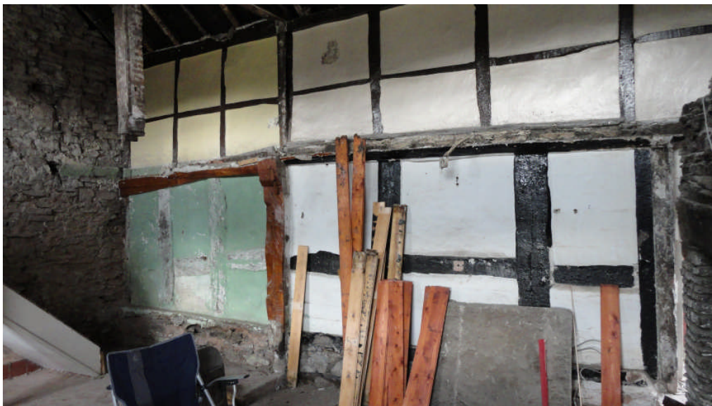
Photo 3: The timber framing in the N wall
