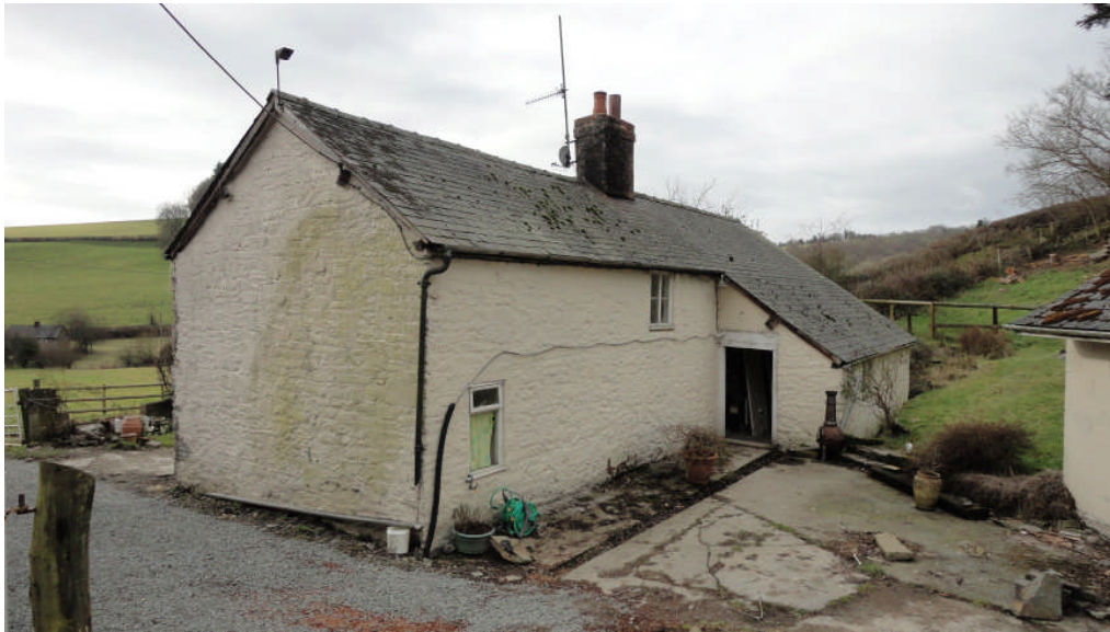
Photo 2: Forest View, showing the outshut and catslide roof, looking SW
