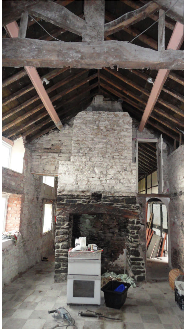
Photo 5: The chimney and fireplace in the E cell, looking W
