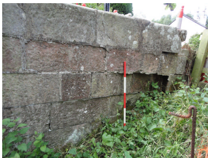
Photo 6: The damage to the northeast wing wall (looking NW)
