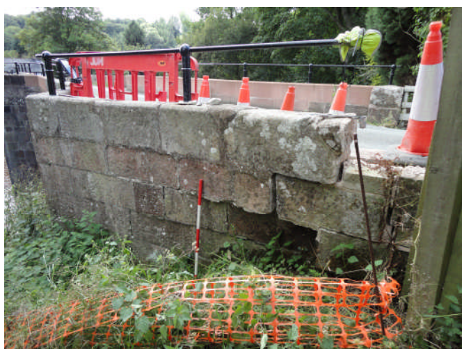
Photo 5: The damage to the northeast wing wall (looking SW)
