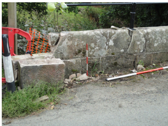
Photo 4: The damage to the northeast wing wall (looking E)
