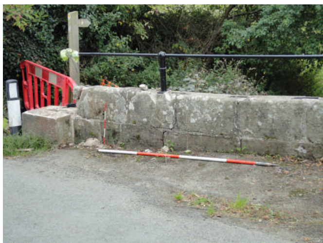
Photo 3: The damage to the northeast wing wall (looking NE)
