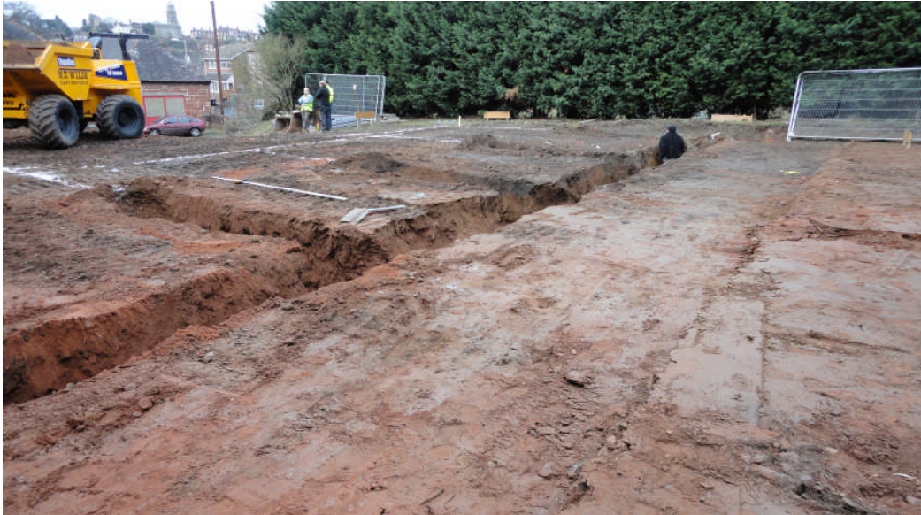
Photo 1: The foundation trenches, looking northwest
