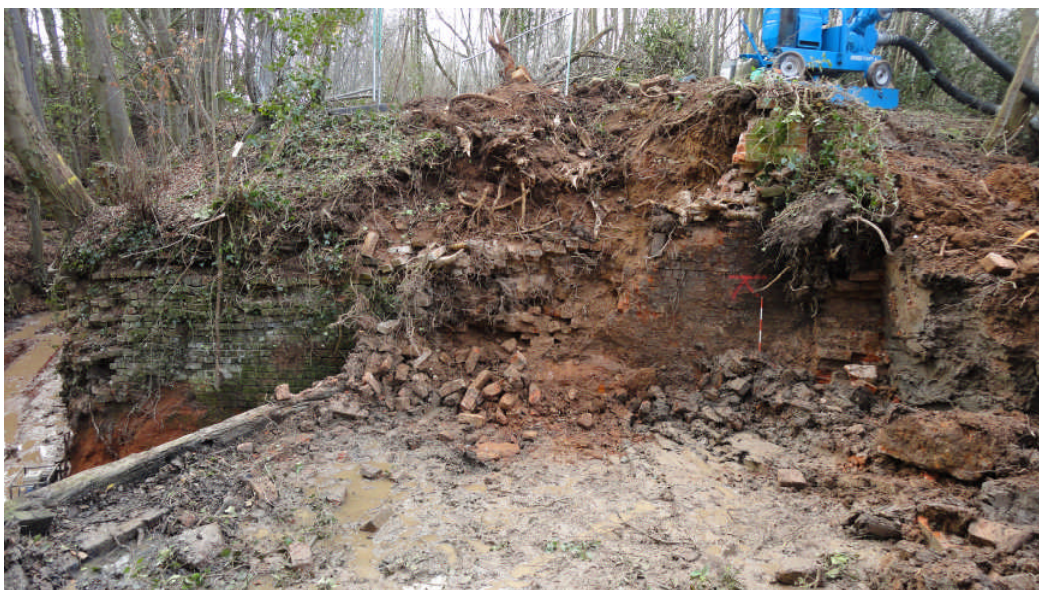
Photo 6: The weir and spillway, looking W, (scale 0.5m)
