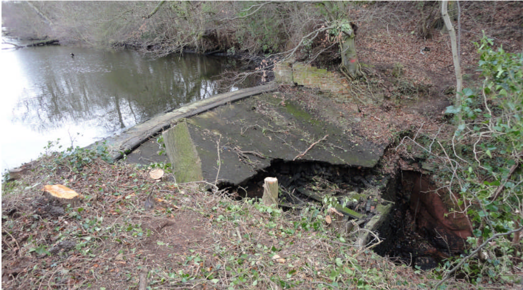
Photo 4: The top of the weir and spillway, looking NE
