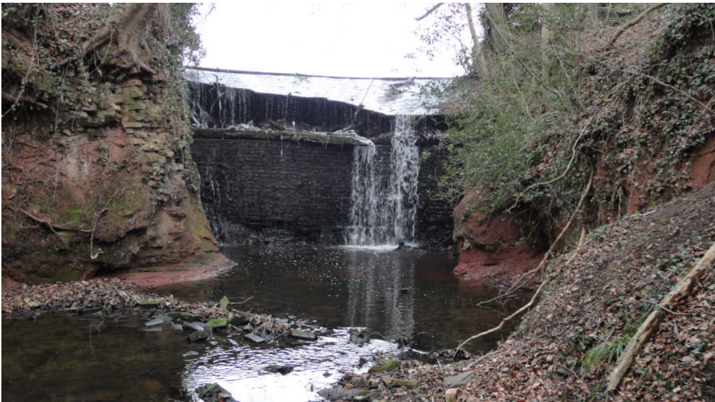
Photo 2: The weir and spillway from below, looking NW
