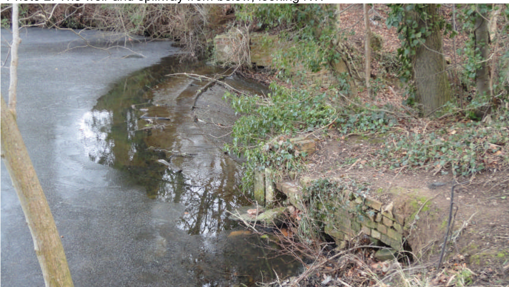
Photo 3: The top of the weir and spillway, looking E
