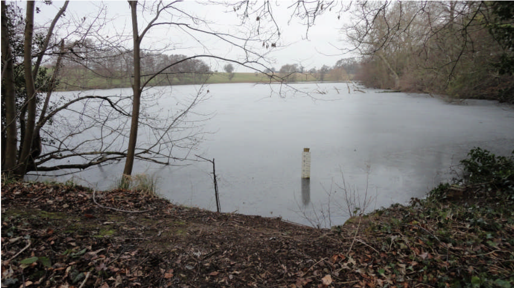
Photo 1: Sunderton Pool from the pool dam, looking N
