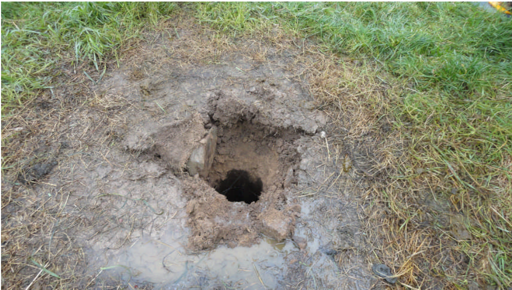
Photo 2: The hole after withdrawing the old electricity pole
