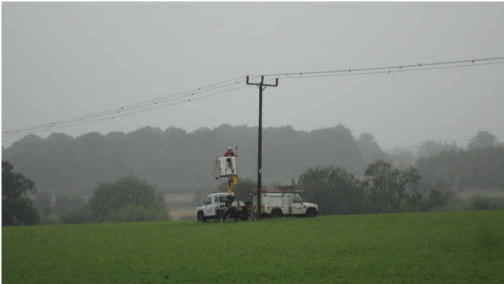
Photo 1: The electricity pole to be replaced, looking NW
