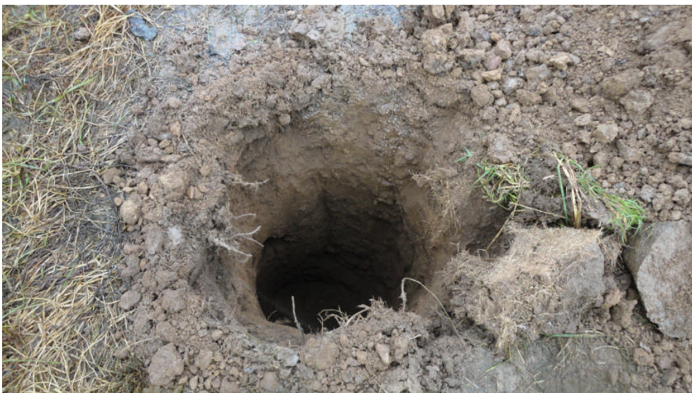
Photo 3: The hole after cleaning with an augur
