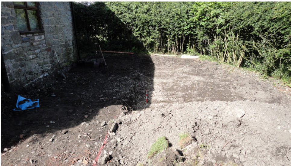
Photo 2: The area of the extension stripped of topsoil, looking W
