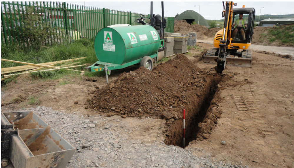
Photo 1: The service trench, looking NE (scale bar 1m)
