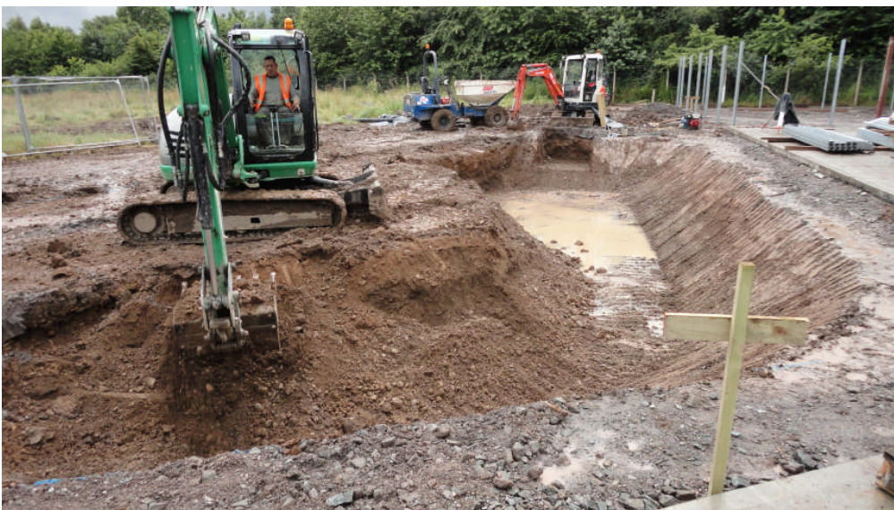
Photo 3: The attenuation pond, looking SE
