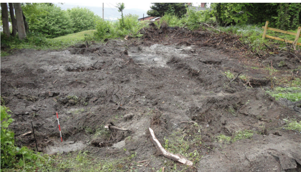
Photo3: The 2013 foundation pits, looking NW, scale bar 0.5m
