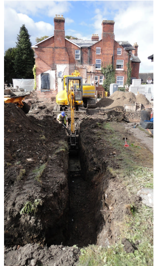
Photo 6: The eastern side of the development, looking W
