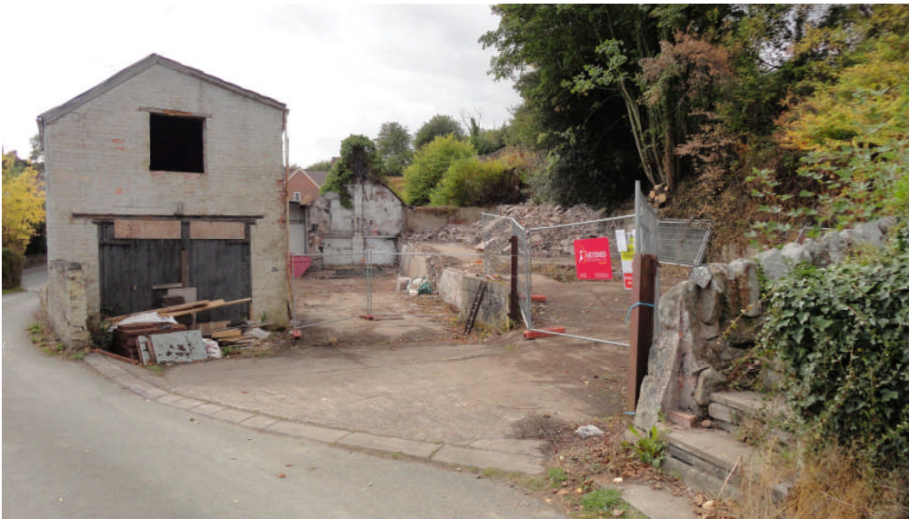
Photo 2: The study area in December 2011 prior to demolition work, looking SW
