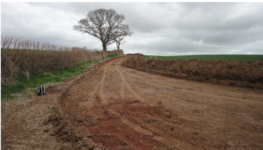
Photo 3: Excavations for the new access track, looking N
