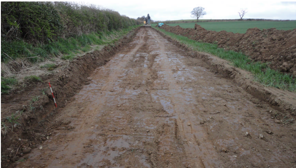
Photo 2: Excavations for the new access track, looking W, scale bar 05m
