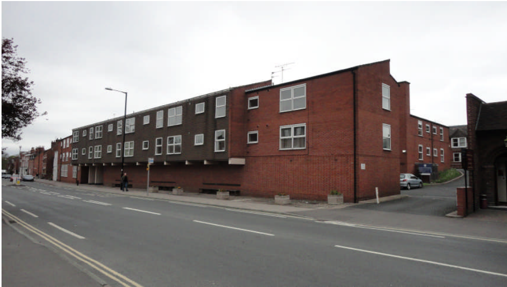
Photo 1: Heath's Houses, looking NW
