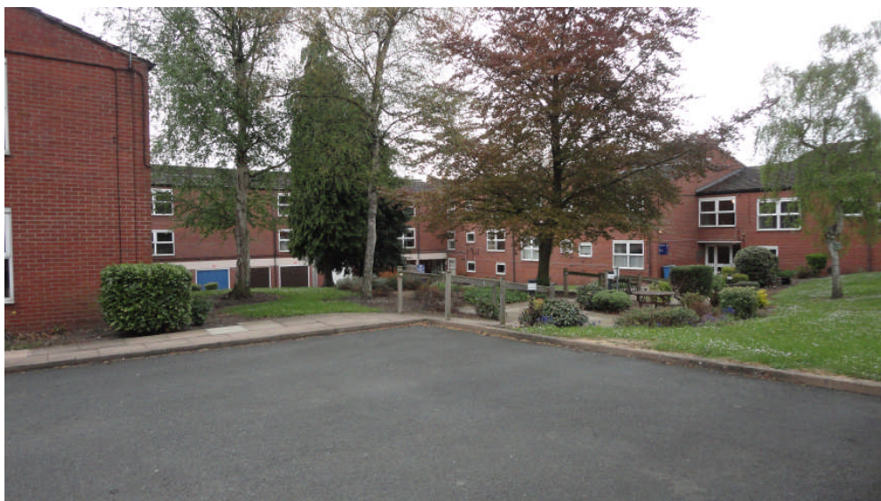
Photo 3: Courtyard and gardens, Heath's Houses, looking SW
