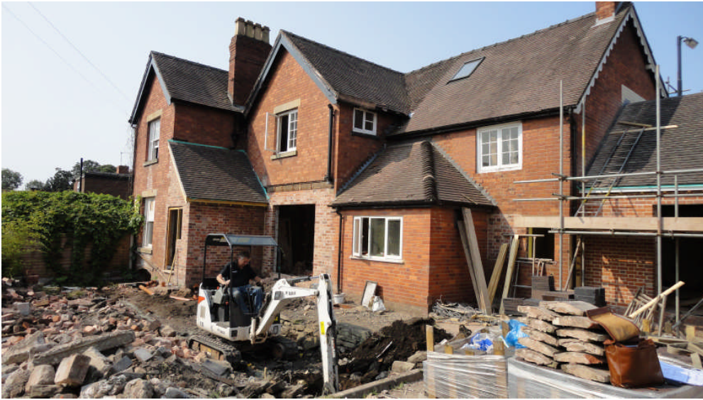
Photo 1: The development site, looking SW
