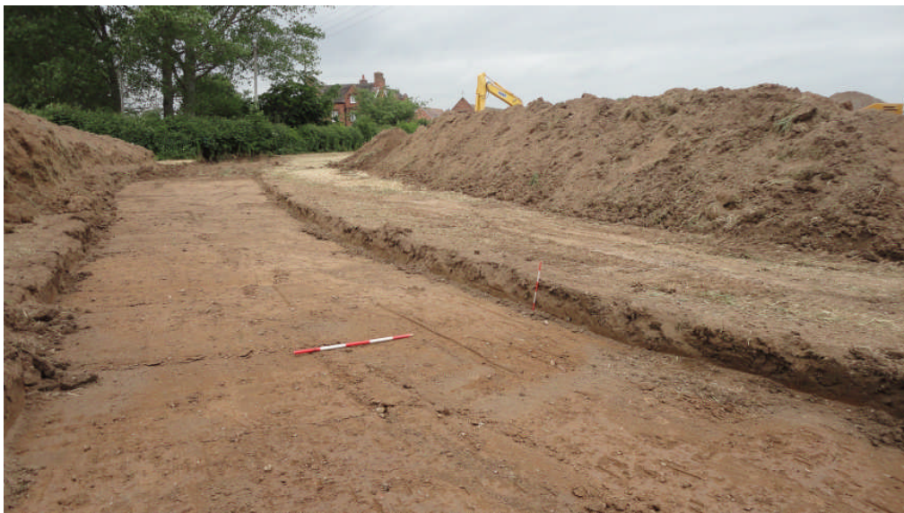
Photo 2: The re-aligned driveway, looking NW, scales 1m and 0.5m
