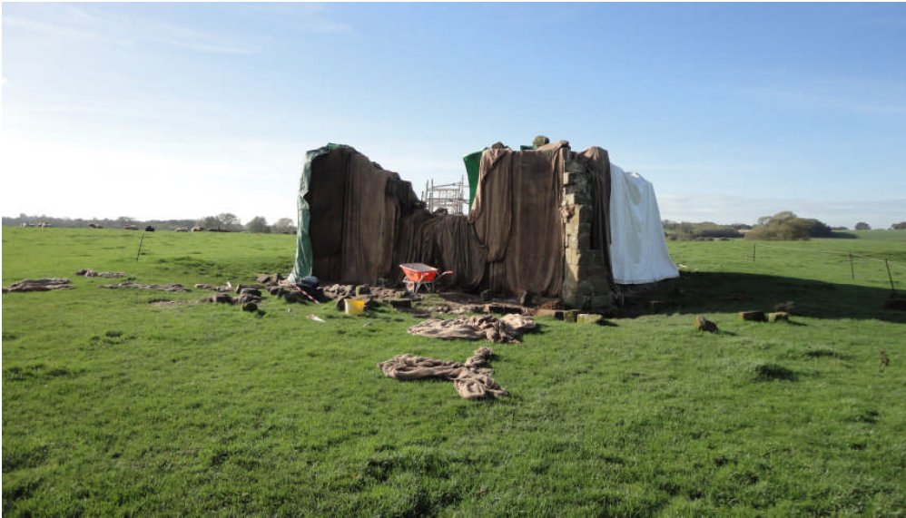
Photo 1: Creswell Chapel during repairs in 2013, looking W
