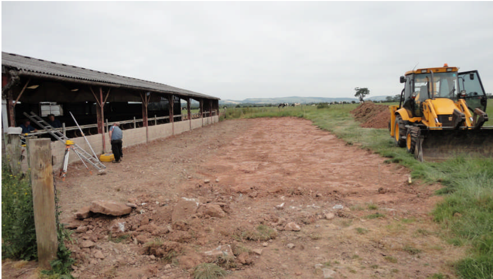
Photo 1: The development site, looking N
