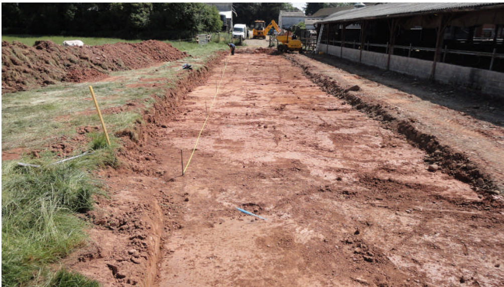
Photo 2: The site stripped of topsoil and overburden, looking S
