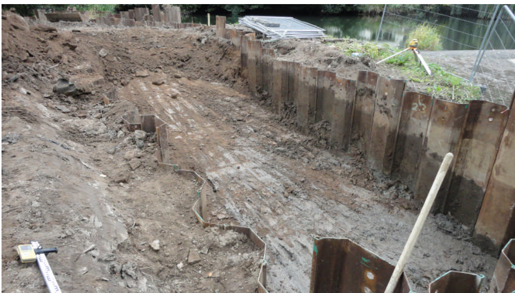
Photo 3: The finished excavations for the main part of the fish pass
