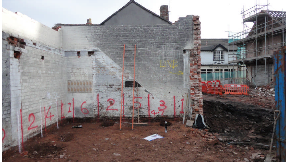
Photo 1: The site at 3-5 Stafford Street, looking SE
