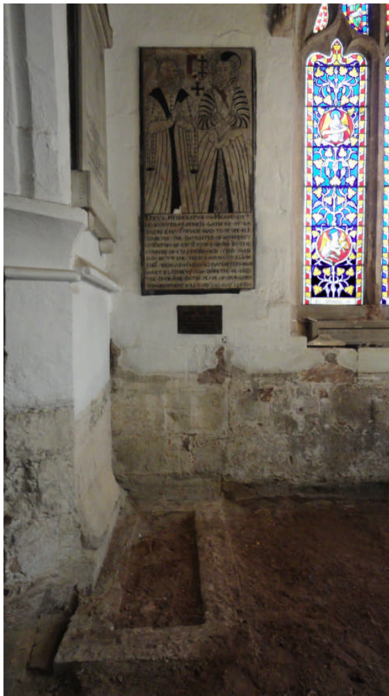
Photo 5: The brick vault and slab to Francis Gatacre, looking E
