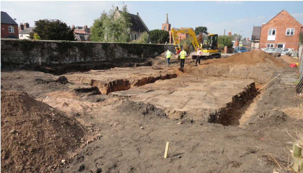
Photo 2: The development site, looking NW
