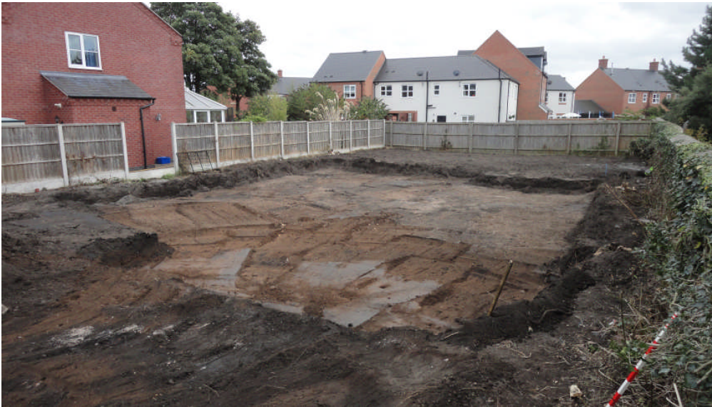
Photo 1: The development site, following the topsoil strip, looking SE
