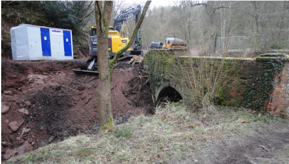
Photo 1: Creating the access into the bypass channel
