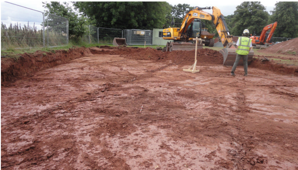
Photo 2: The topsoil strip for the new car park, looking E
