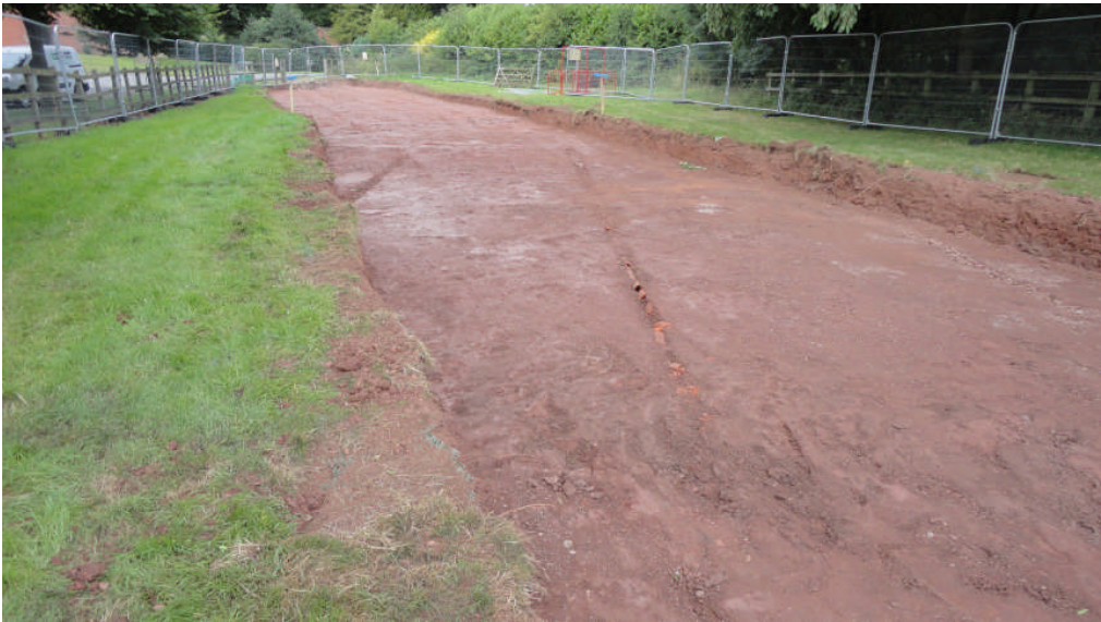
Photo 1: The topsoil strip for the new access, looking W
