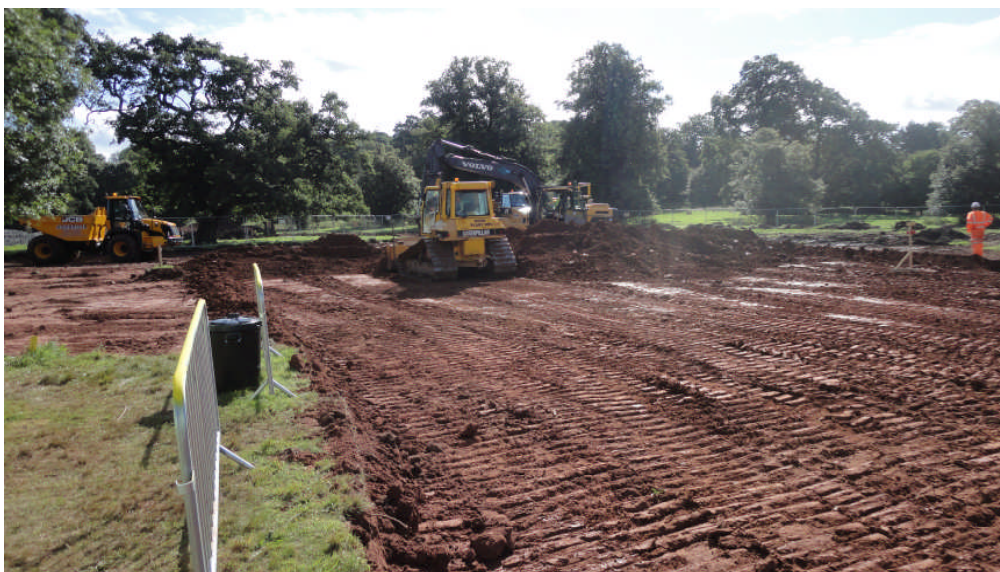
Photo 3: The topsoil strip for the new overflow car park, looking SE
