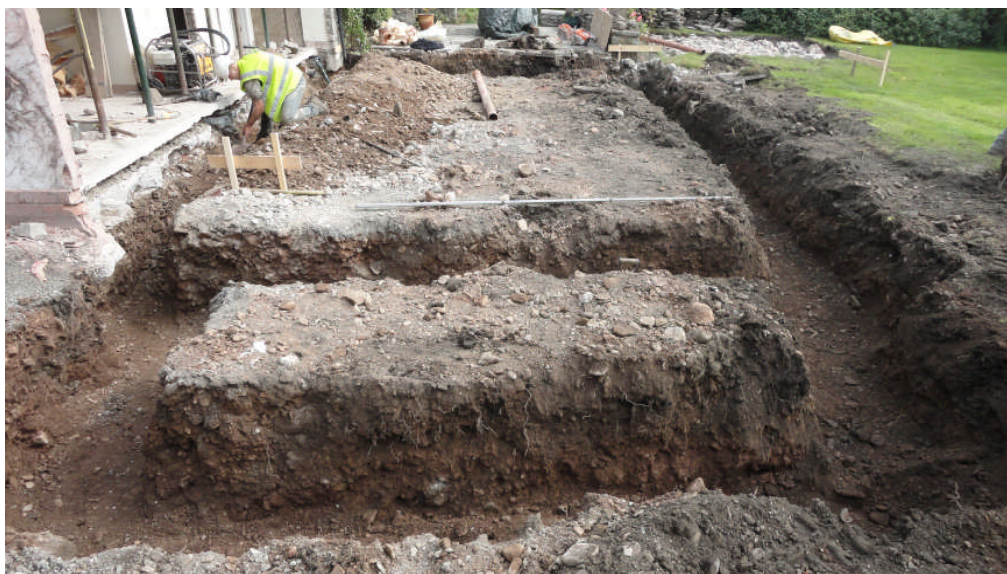
Photo 3: The foundation trenches for the new extension, looking E.
