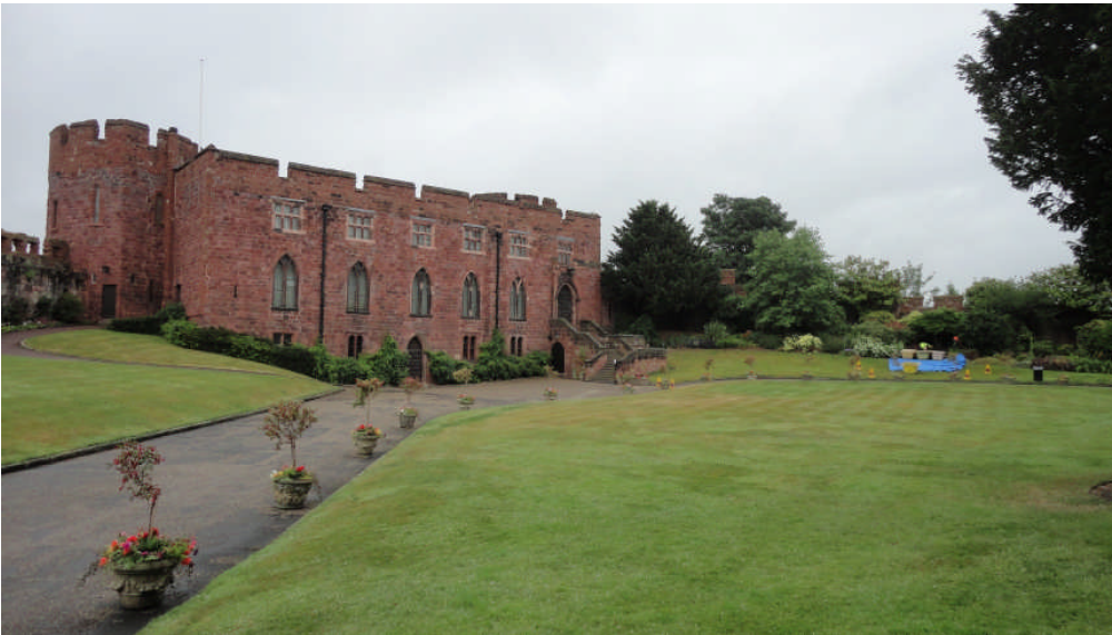
Photo 1: The location of the foundation pit (centre right), looking NE across the castle inner bailey.
