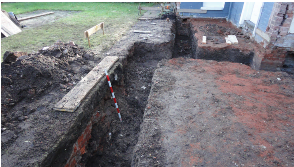
Photo 3: The foundation trenches, looking S; scale bar 1m
