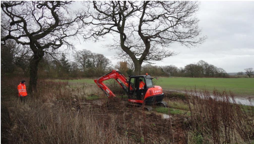
Photo 1: The location of the new ponds, looking NE
